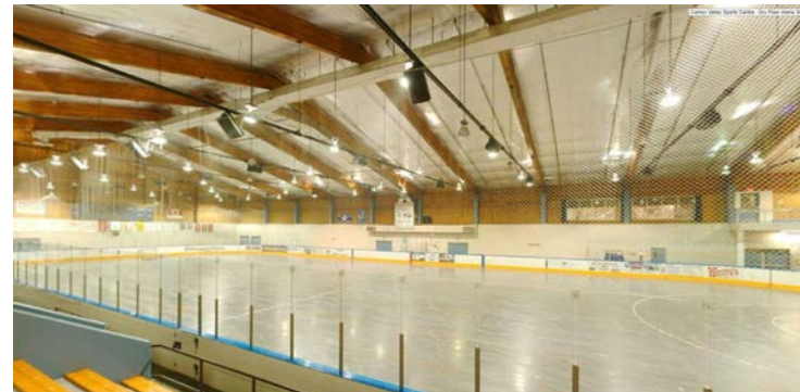
Photo 3 - Arena 1 Interior facing North
