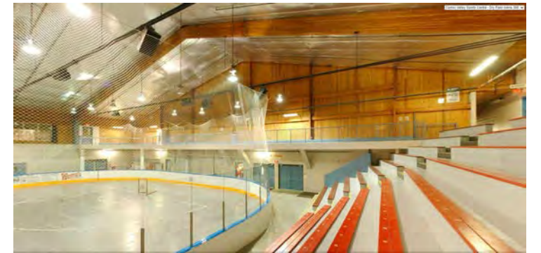
Photo 4 - Arena 1 Interior facing West
