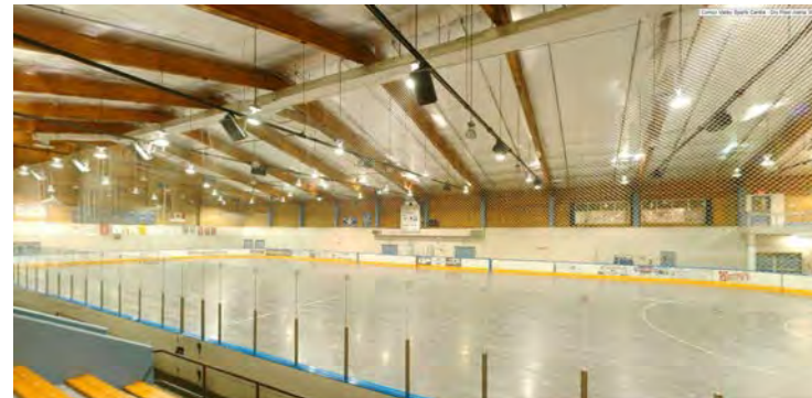
Photo 3 - Arena 1 Interior facing North
