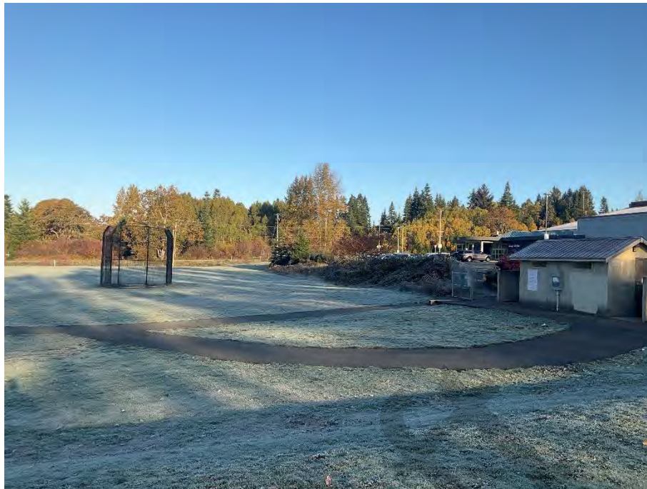
Photo 19. Area 5: View of discus cage to the left and maintenance building to the right.
