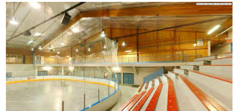
Photo 4 - Arena 1 Interior facing West
